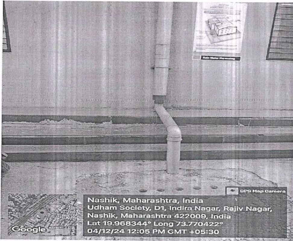
Rain water harvesting system board
